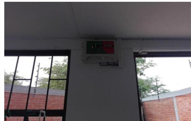
PANEL ENERGIZADOR PAR CERCA ELECTRICA 1200V, 1.2 JOULES, INCLUYE BATERIA 12 V 7AH
